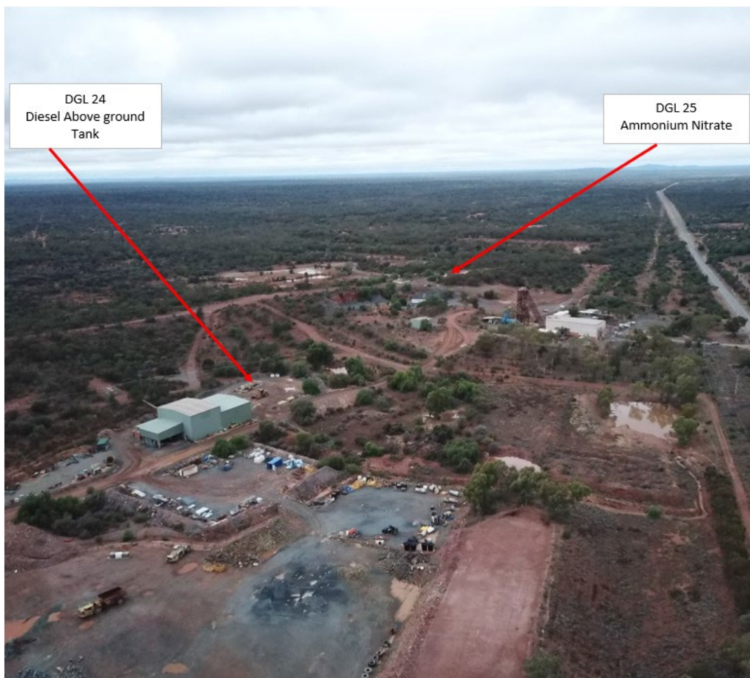
Figure 4: New Cobar Dangerous Goods Locations
