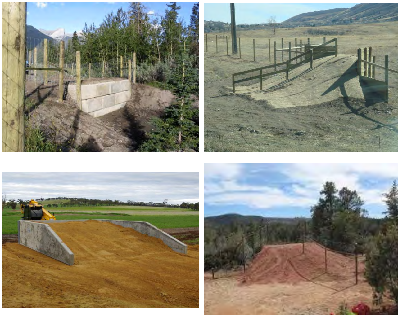
Plate 3: Examples of wildlife escape ramp designs.
