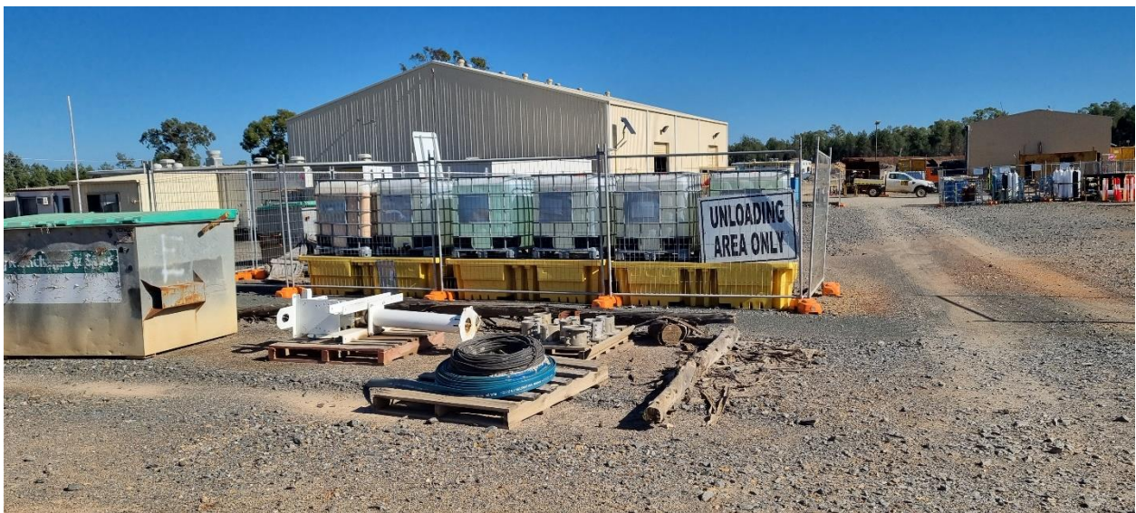
Photograph 2 – Typical storage of process plant chemicals (no cyanide) at the Hera site
