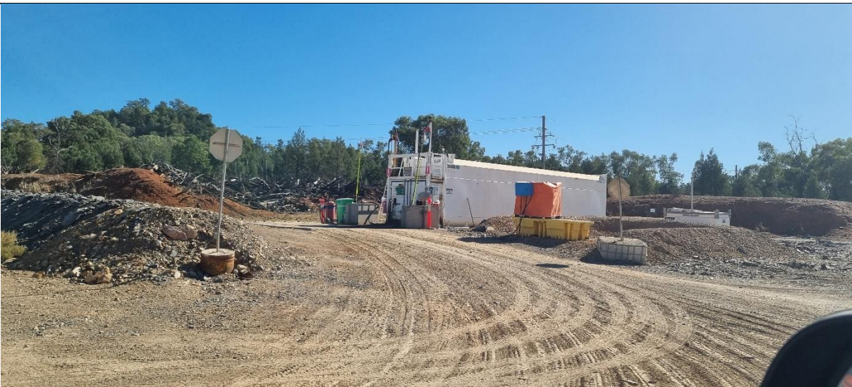
Photograph 3 – Bulk Fuel Storage at the Hera Site
