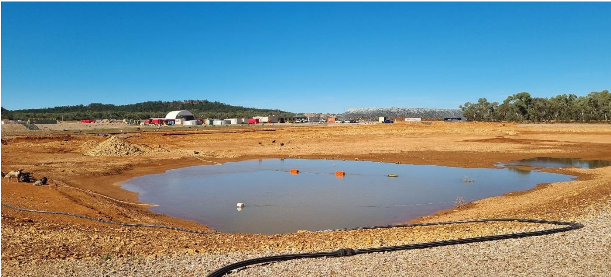
Photograph 17 – Federation surface works (surface water storage dam in foreground)
