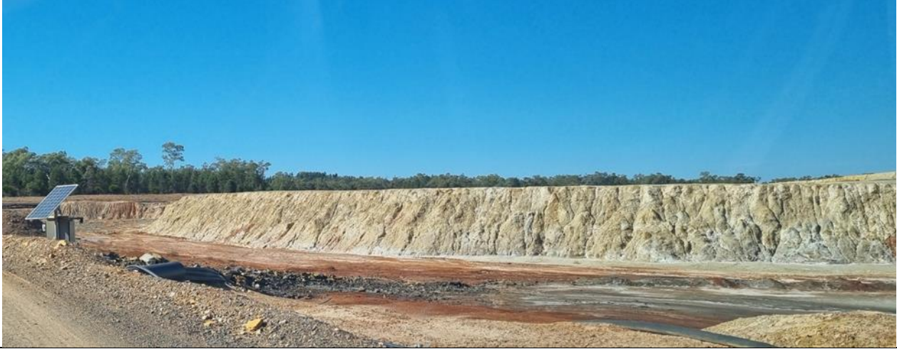
Photograph 7 – Hera TSF taken from the Hera access track
