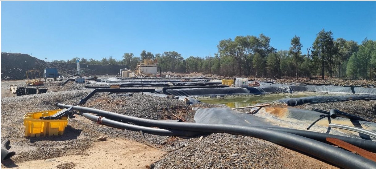
Photograph 4 – Hera process water treatment ponds
