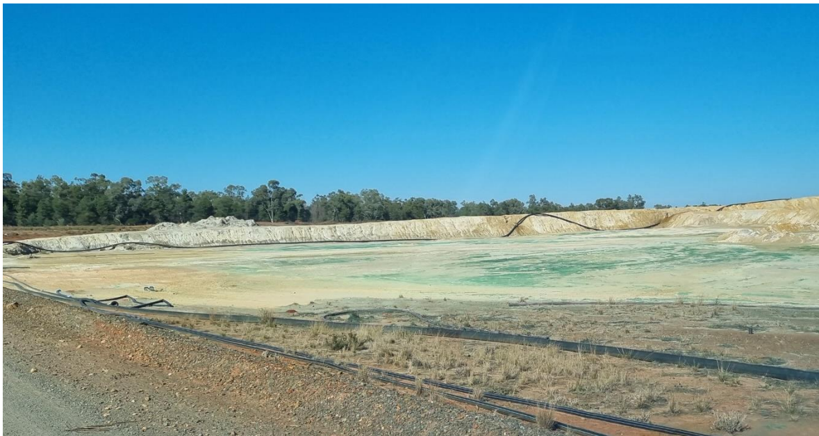
Photograph 8– Hera TSF showing (green) dust suppression binder
