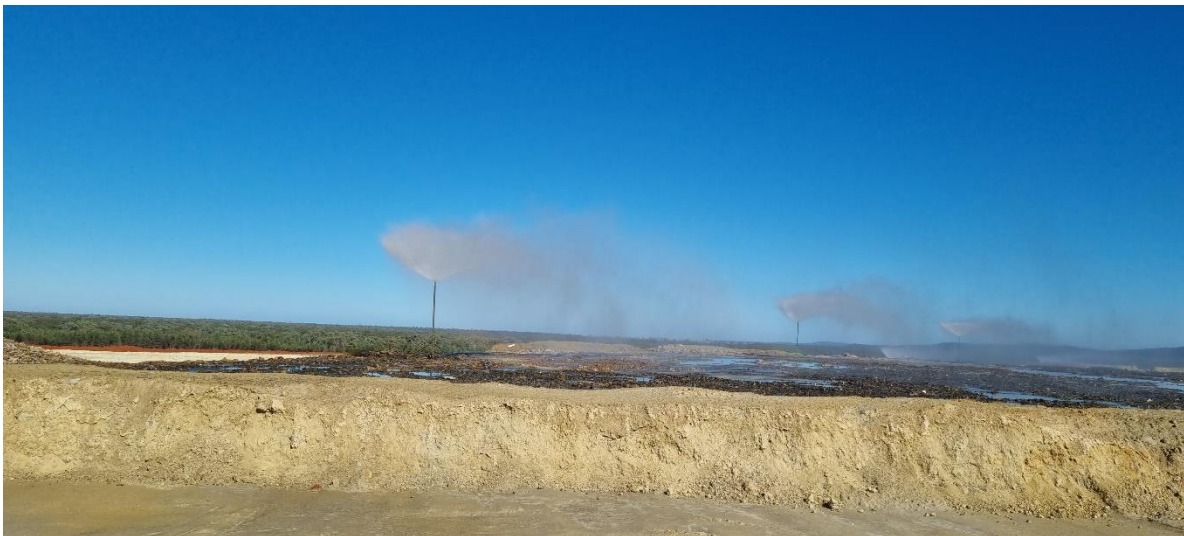
Photograph 9– Hera TSF dust suppression / excess water evaporation sprays
