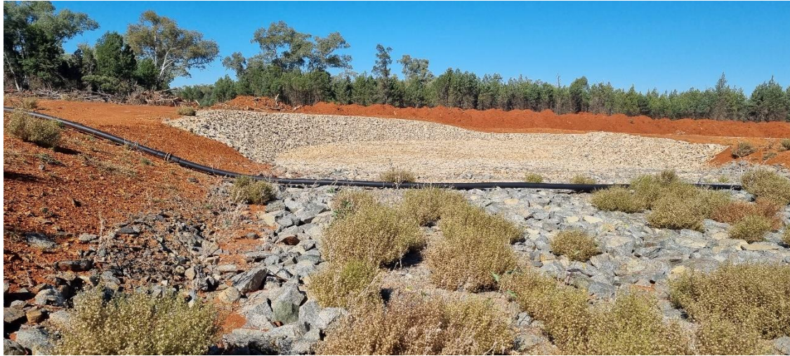
Photograph 10 –Hera TSF discharge channel stabilisation
