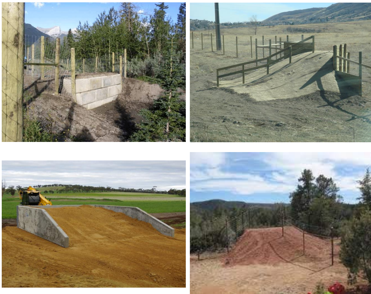
Plate 3: Examples of wildlife escape ramp designs.
