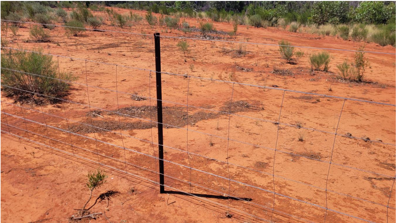
Plate 1: An appropriate exclusion fence design without barbed wire.
