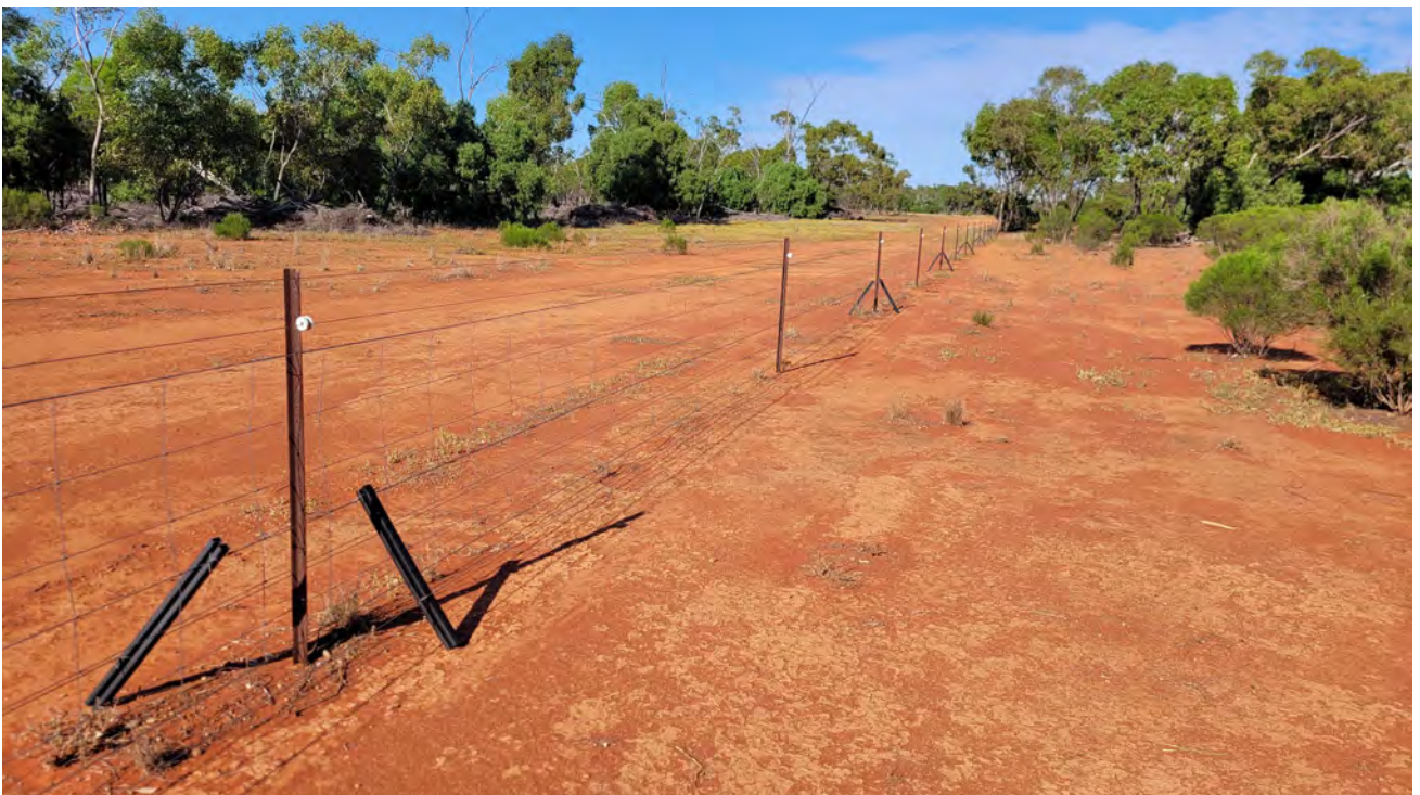
Plate 2: An appropriate exclusion fence design using electrified wire.
