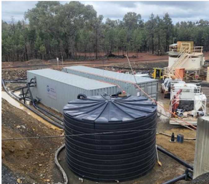
Water Treatment Plant and location of Back Tank east :
