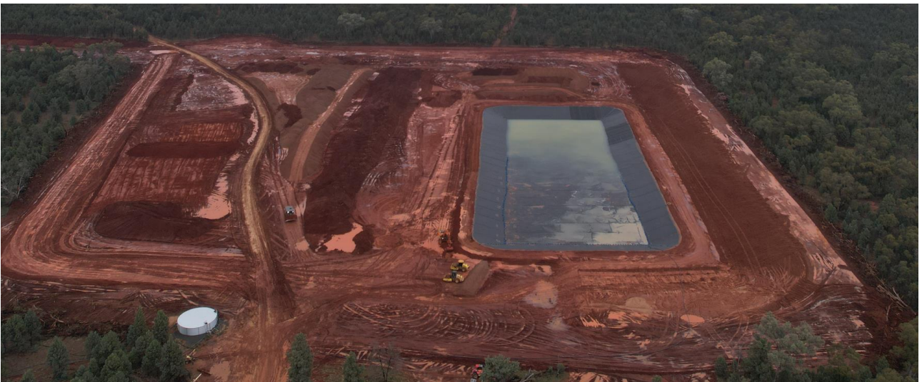
Figure 2: Completed 30ML lined sump dam within the perimeter of the larger 230ML water management dam.
