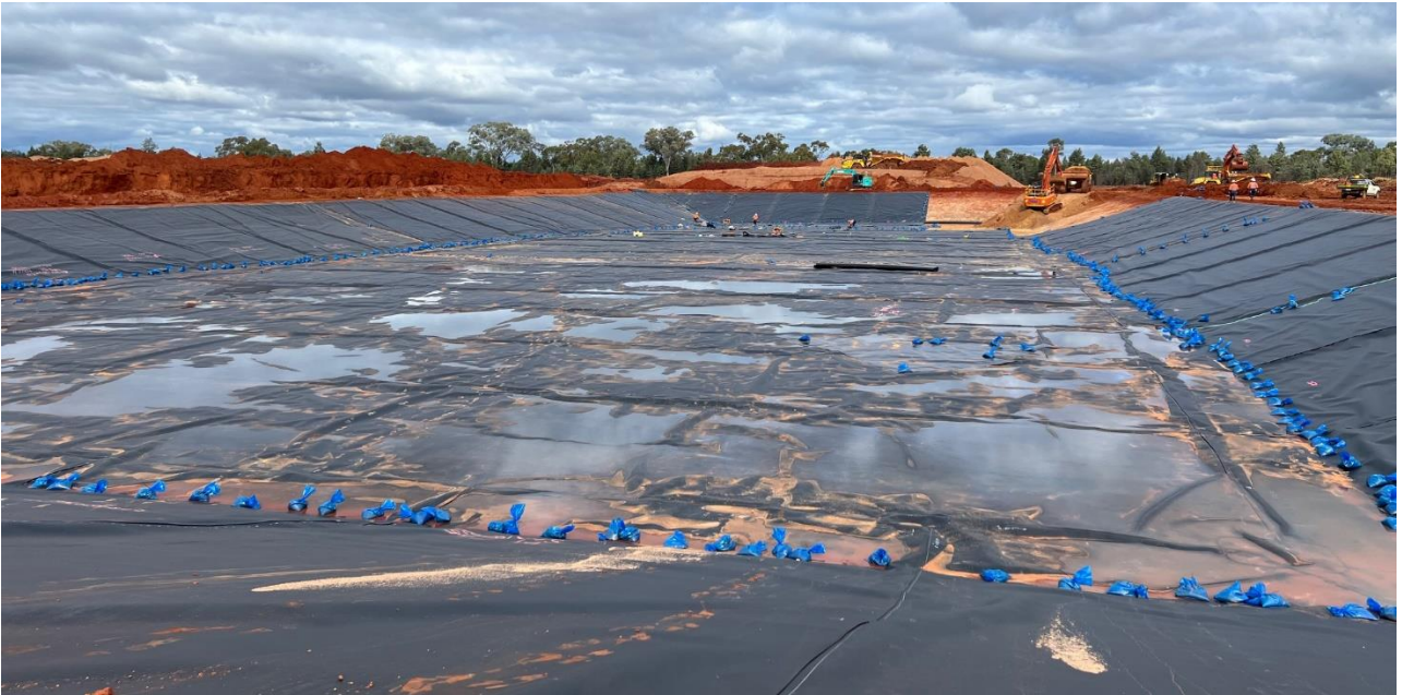
Figure 1: Lining of 30ML sump dam nearing completion.
