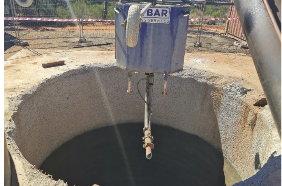
Shotcreted Return Air Rise
