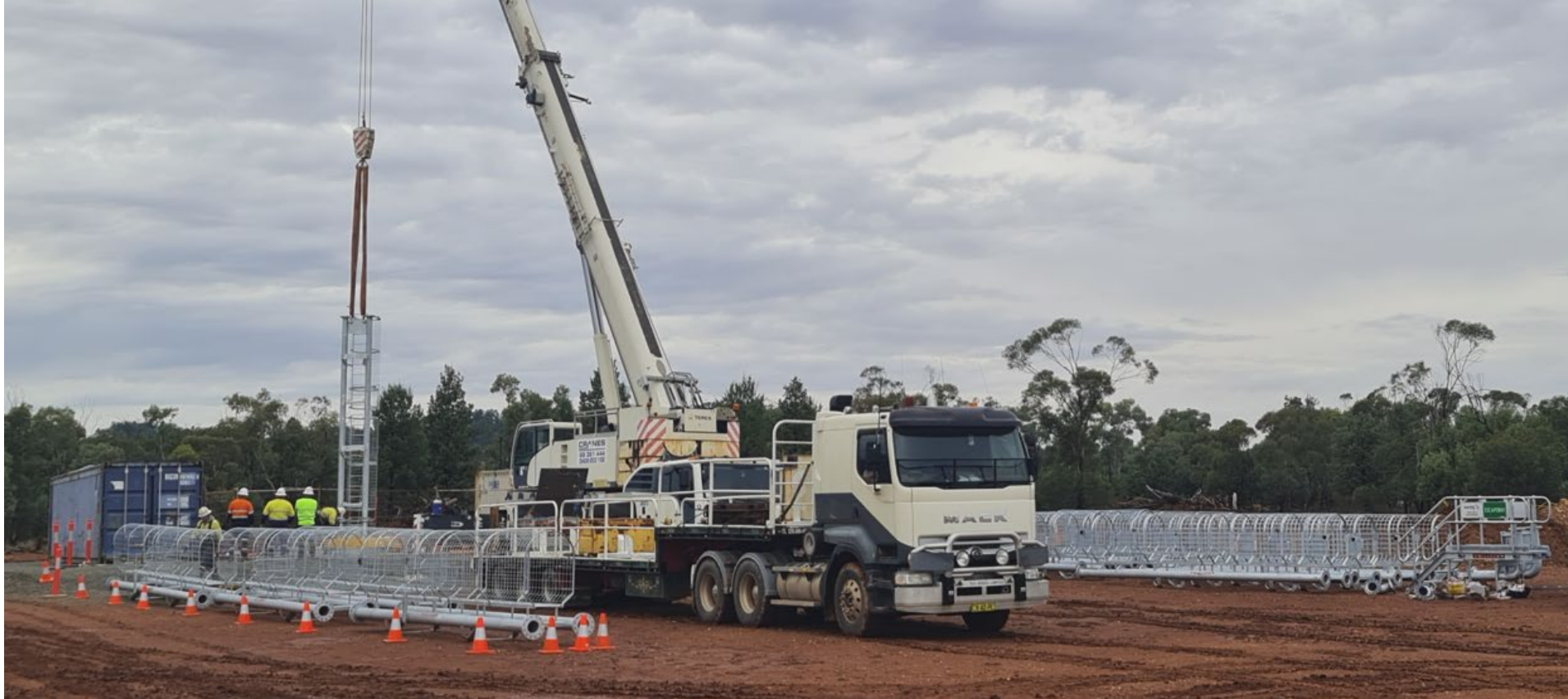
Surface to 1230 Level Ladder Installation
