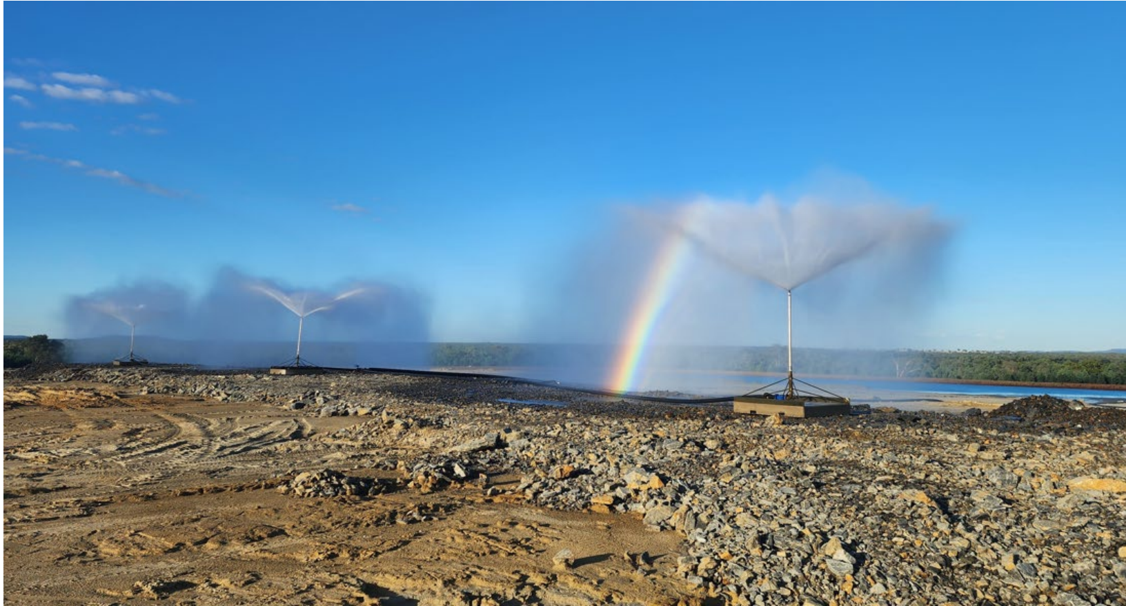
Evaporators/misters on TSF in operation
