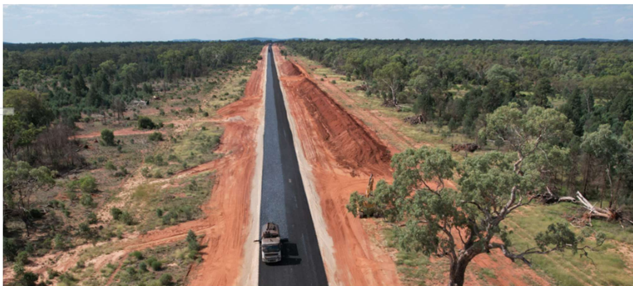
Figure 4: Road sealing works along the Burthong Road.
