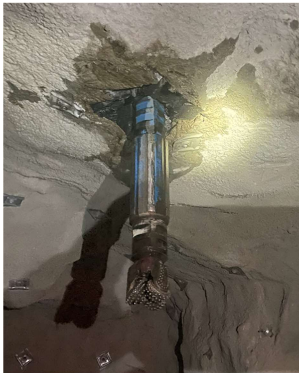
Figure 2: Pilot hole breakthrough
