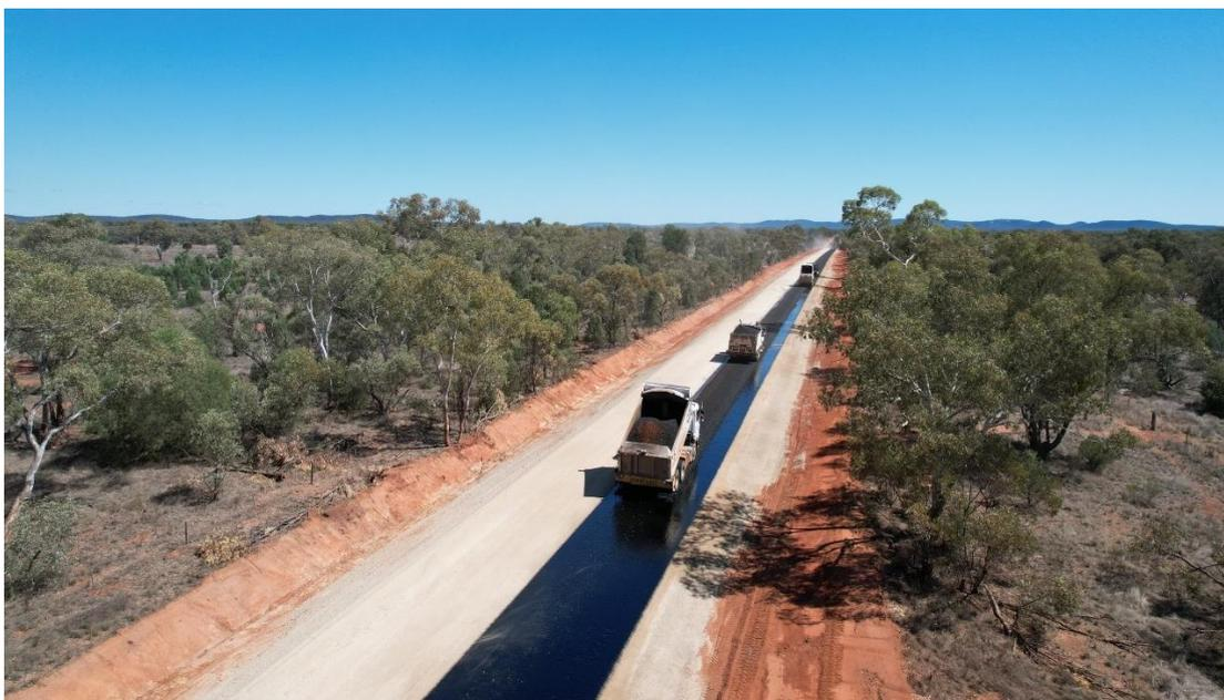
Image 1: Burthong Road sealing works in progress.
