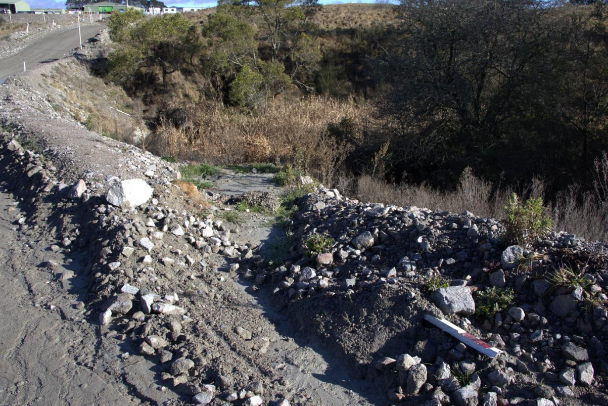
Photograph 7 - Drainage from Spring Creek Crossing
