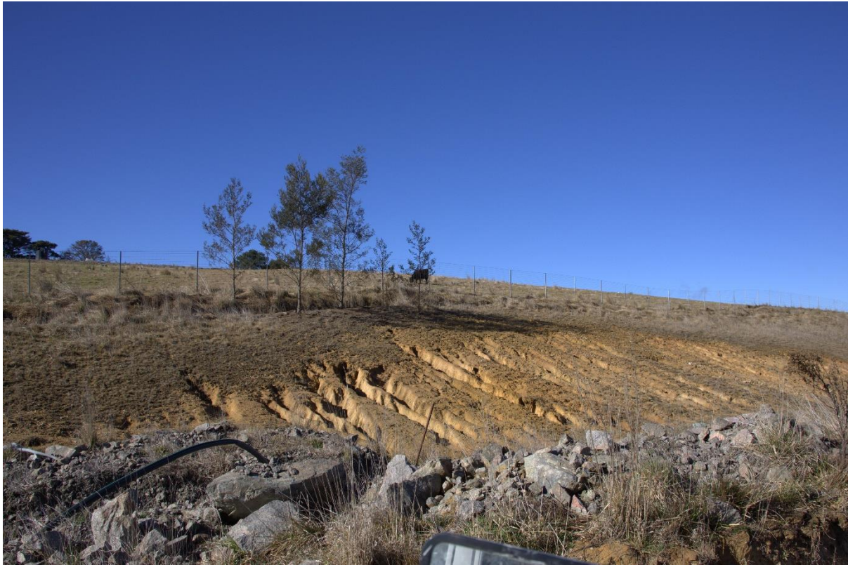
Photograph 5 - Erosion of the TSF Clean Water Diversion
