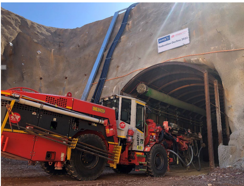
Figure 1: Jumbo tramping into the portal at the Federation Project
