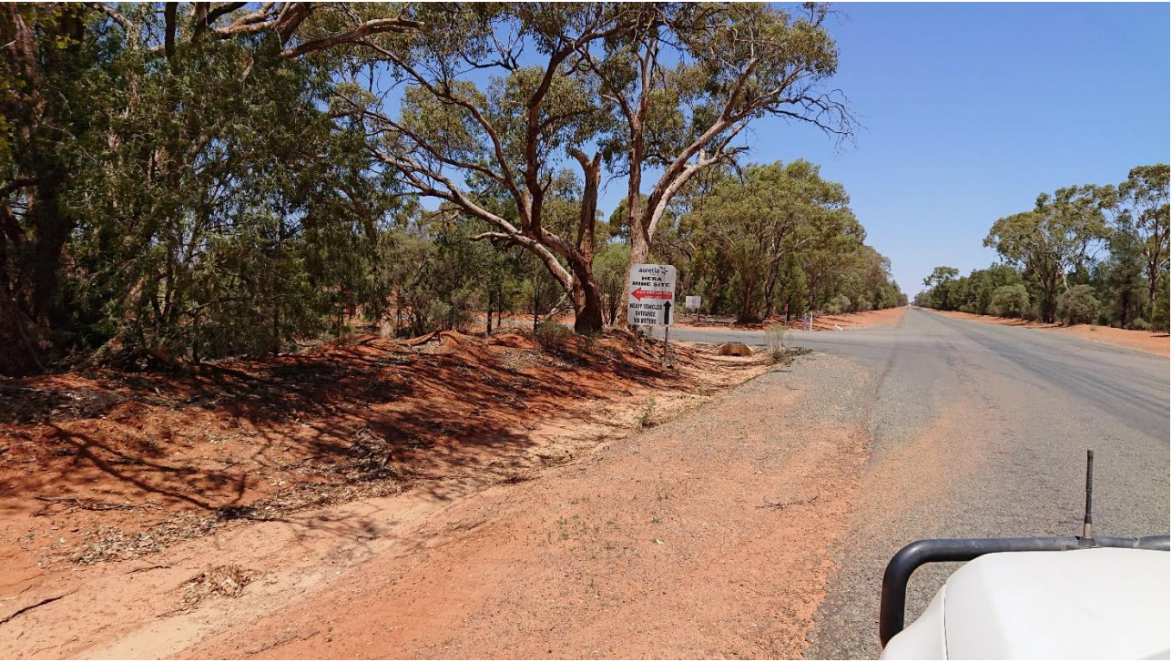
Photo # 7 - Light Vehicle Access Intersection
