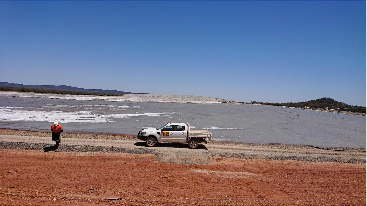
Photo # 6 - Tailings Storage Facility
