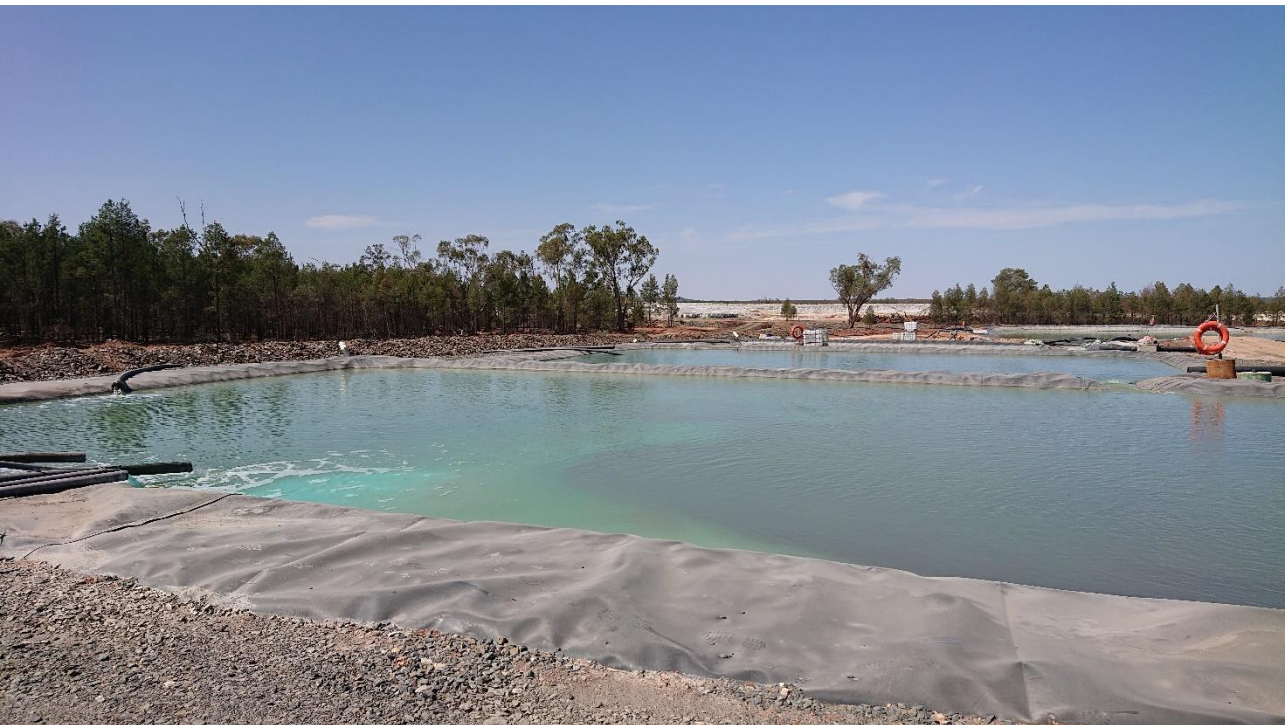
Photo # 4 - Process Water Management System
